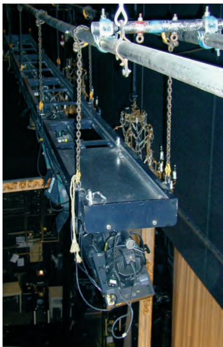
A focusing trolley at the near end of the suspended track which forms part of the touring lighting rigs. The lighting technician lies on the trolley and can reach and set the lights beneath.
